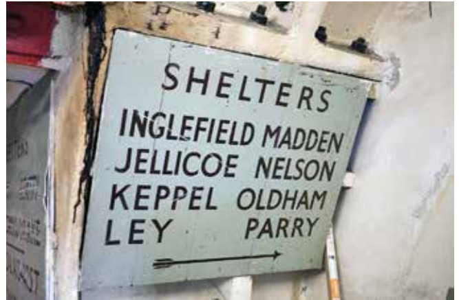
Each tunnel was divided into 4 sections with connecting doors between them. Each section was given a name. At Clapham South they were all naval commanders. The northern entrance sections (i.e. those accessed directly from the northern lift without crossing to the other side) were named: Fremantle, Beatty, Evans, Anson, Nelson, Jellicoe, Madden and Inglefield while those accessed from the southern entrance were: Grenville, Hardy, Drake, Oldham, Keppel, Parry and Ley. Many of the signs are still in place throughout the shelter. Photo Konstantin Binder
